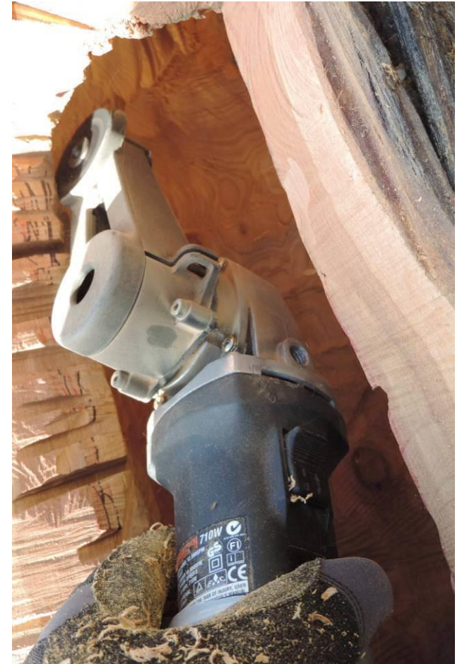
Figure 43. Once the cavity has been sufficiently enlarged the smaller Arbortech wheel can be used to smooth any rough edges and for finer scale carving and contouring.
