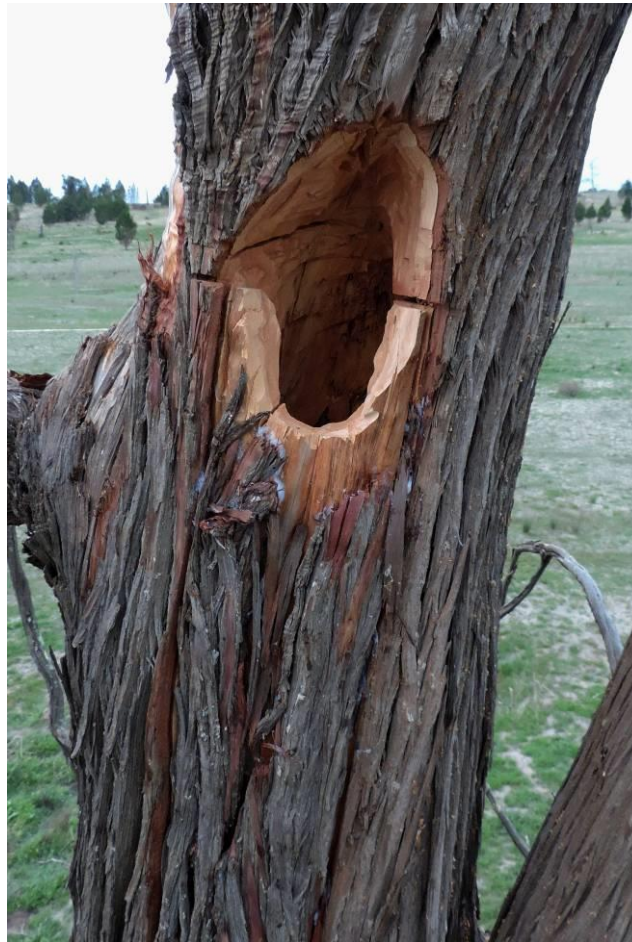
Figure 16. After replacing the face plate, the bark layer is glued and screwed back in place to cover the tech screws.
